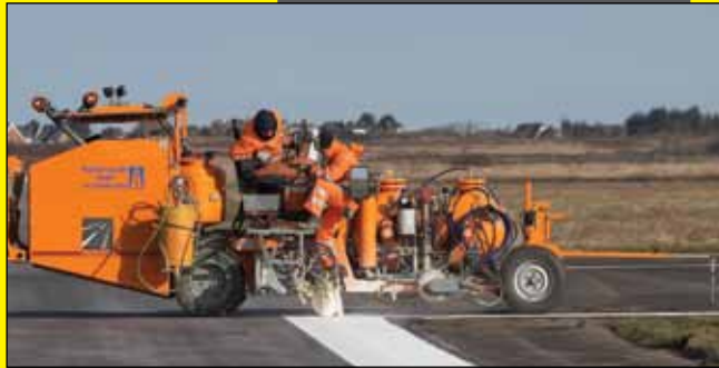
Airport Marking Machine With Wide White Line
